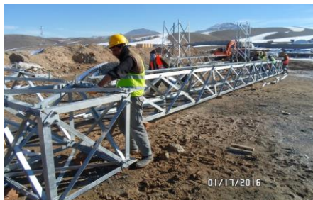
Workers install equipment to erect an electricity tower.
