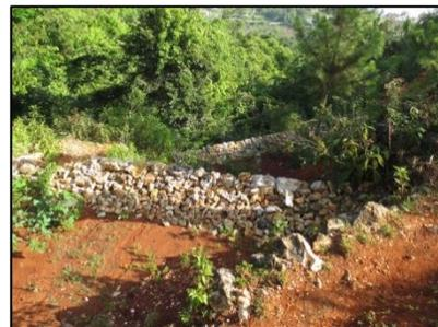
*This newly built gully plug helps slow the rate of water and debris flowing down Millet Ravine.*
