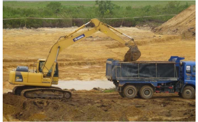
Contaminated soil excavation in the storage area (Photo: USAID)
