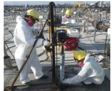
Drilling for samples (Photo: CDM Smith)
