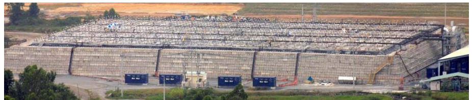
Thermal treatment structure in operation
