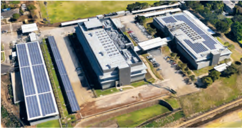
At its office compound in Pretoria, South Africa, USAID has installed solar panels to reduce its energy consumption-related carbon footprint and to increase its climate resilience and energy security, especially as South Africa continues to implement rolling blackouts due to energy shortages. PHOTO: USAID
