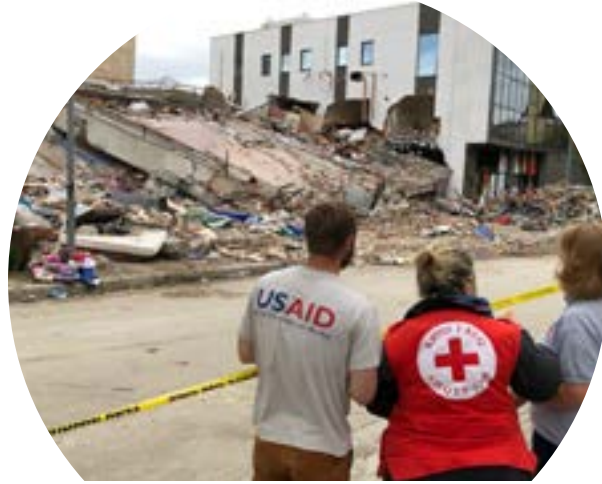
In response to an earthquake in Albania in November 2019, BHA deployed a team of USAR coordination and engineering experts to support the government in damage assessments. Photo courtesy of U.S. Embassy in Albania
