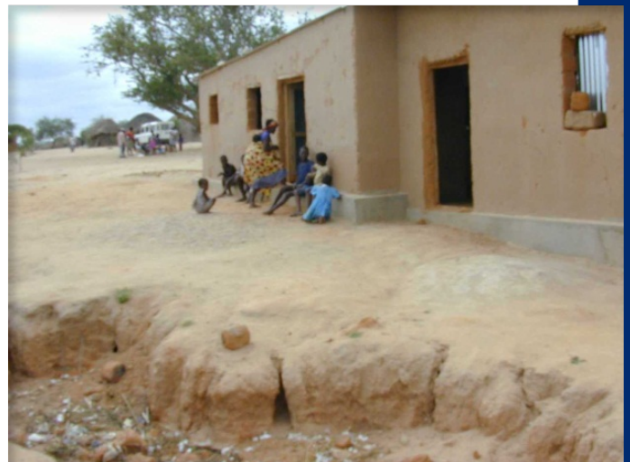
Clay borrow pit (foreground) for health clinic construction with accumulated medical waste in Sumbe, Angola.
