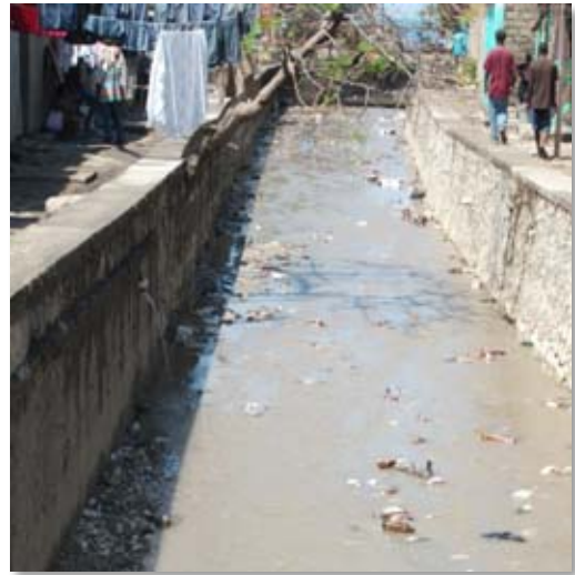
A waterway is visibly contaminated with waste.
