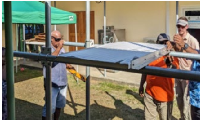
VDAP engineer Aaron Rinehart describes solar panel attachments to MMERE staff during a station demonstration. Photo courtesy of Rowdy LaFavers, USGS.
