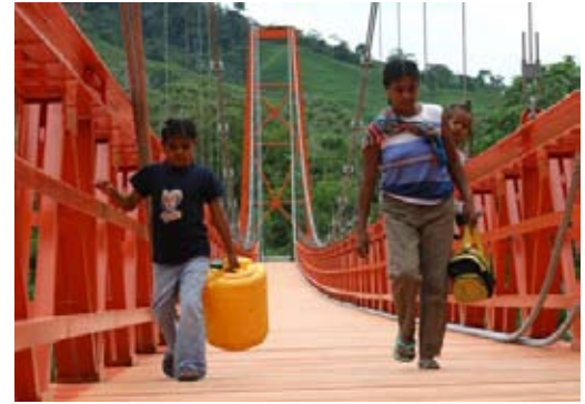
This bridge in Uchiza, San Martin department, was built by USAID to support the surrounding communities' transition to a licit lifestyle.
