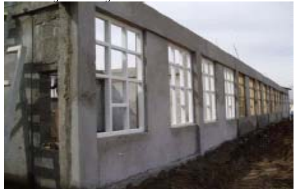
Installation of exterior windows at Kabul school site.
