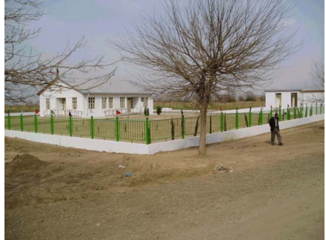
Completed clinic in Kabul province.
