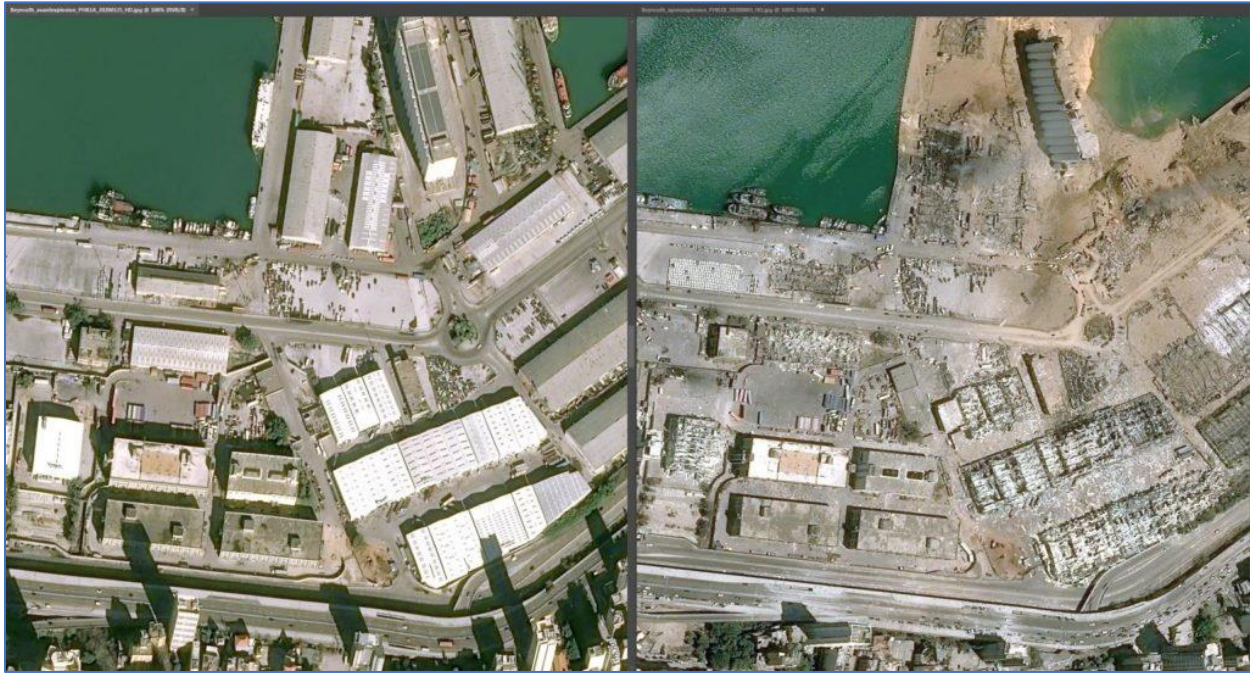
Figure C.2 - POB Free Zone before and after the August 4 Explosion
